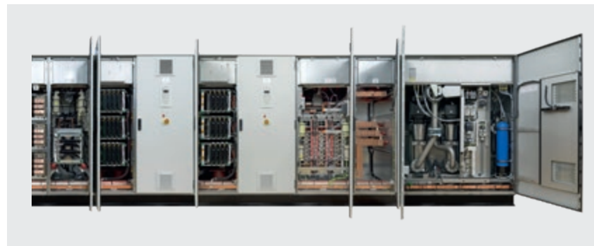
IGBT modules of ABB's grid emulator in operation at Fraunhofer IWES
