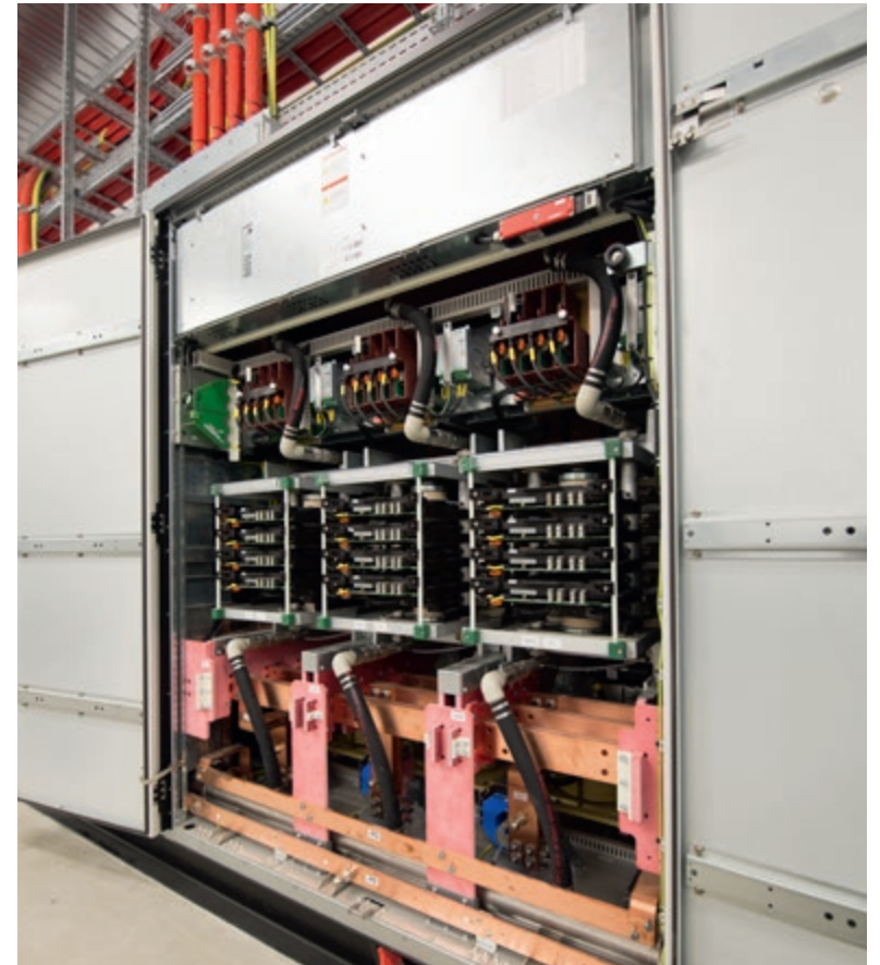
Converter system for grid emulation at the DyNaLab
