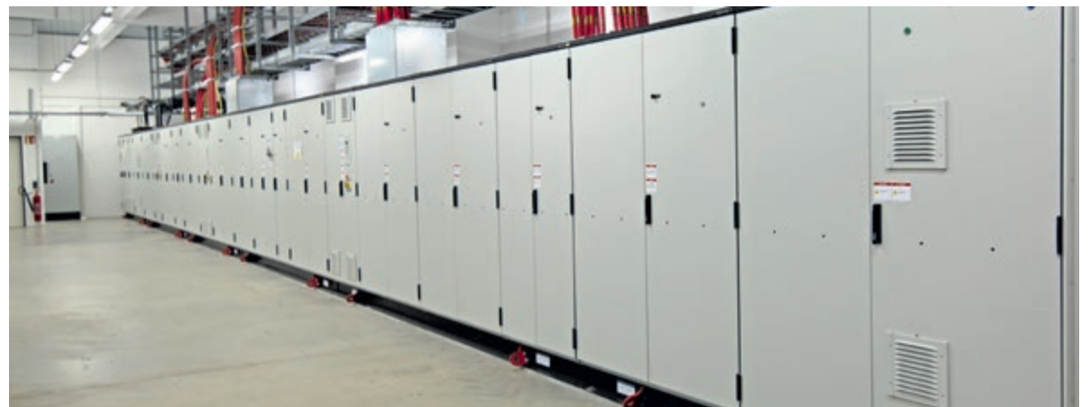
Converter system for grid emulation at the DyNaLab
