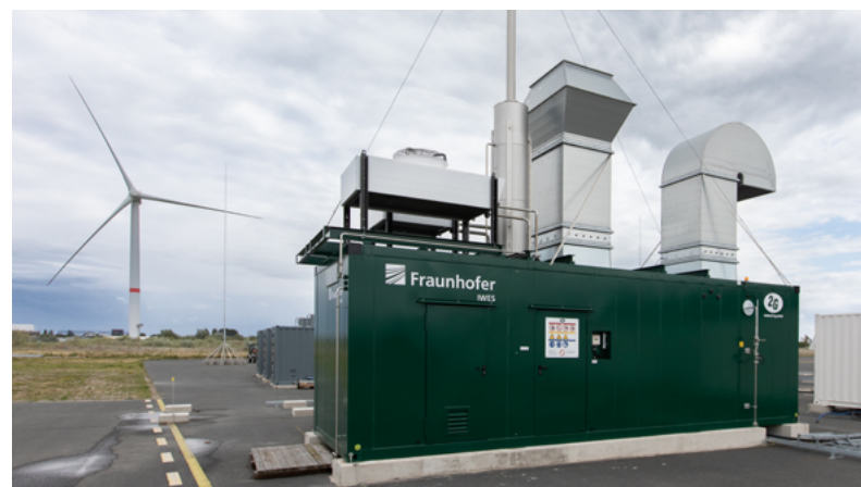
Hydrogen CHP at the HLB testing area with the AD8-180 offshore wind turbine prototype in the background.
